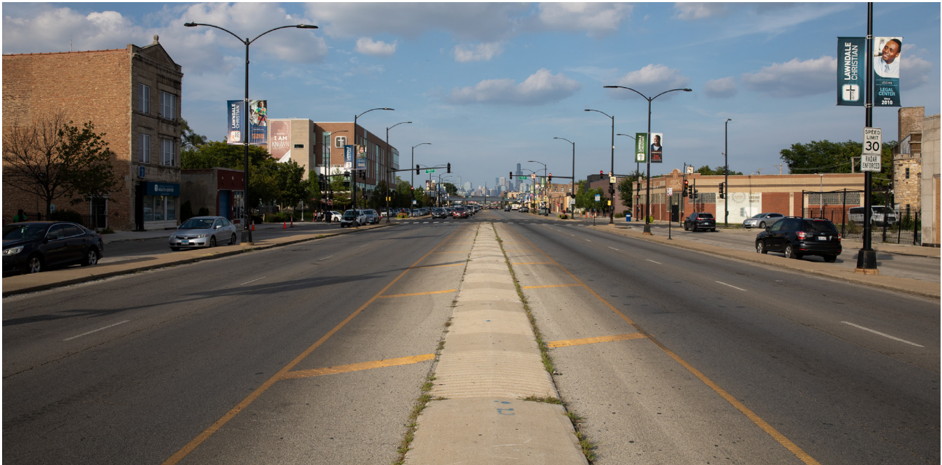
Photo 15. Limited trees and expansive swaths of concrete across Ogden Avenue may lead to increased flooding
